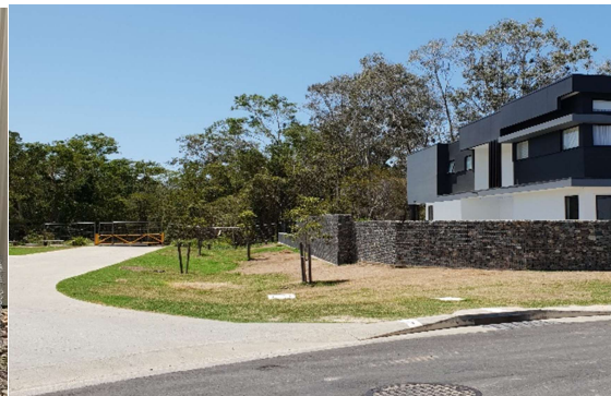
Gabion Fence Using Prophet Mine Rock
